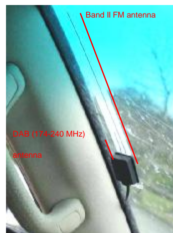
Figure A.3.2.1-9: the Pure Highway's dedicated antenna
